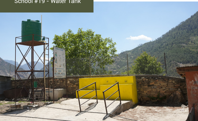
School #19 - Water Tank
